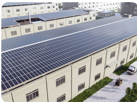
Flat-to-pitched Roof Conversion
