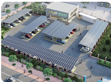
PV Charging Carport With Storage
